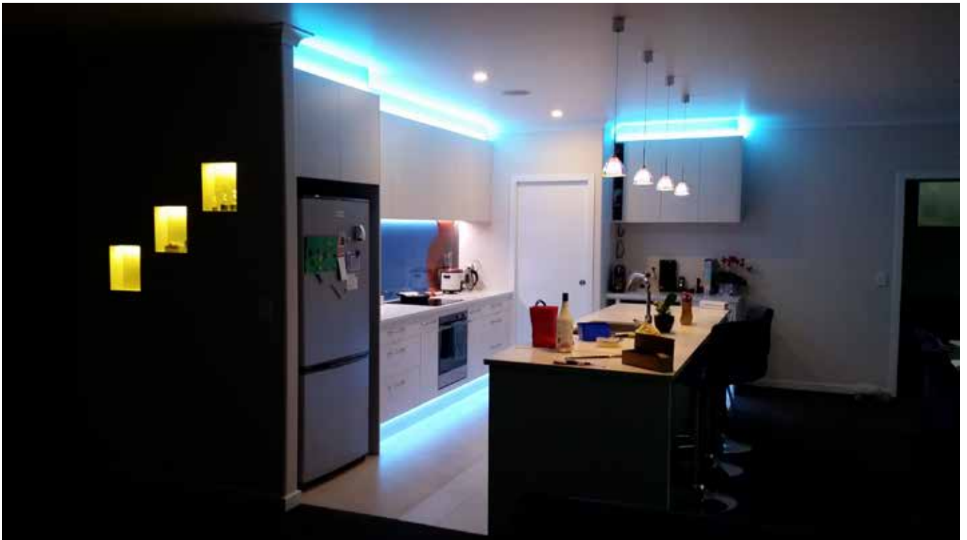
RGBW Strip Light in kitchen bulkhead, splashback, and toekicks
