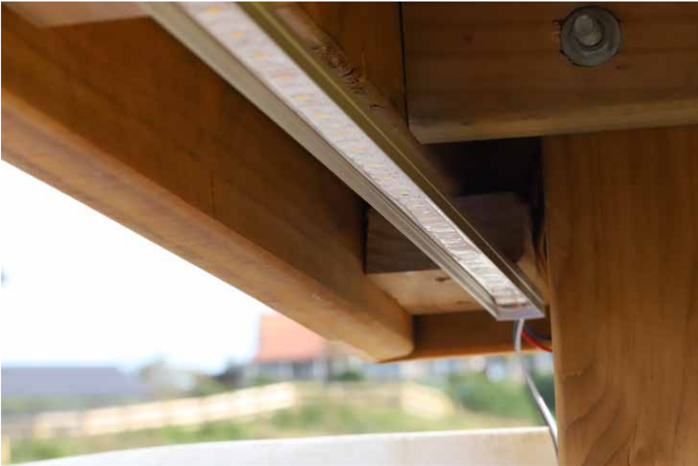
RGBW Strip Light in channel under deck seating
